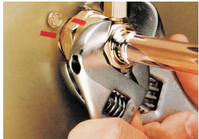
Rotate Swivel Nut ¼ Turn More
