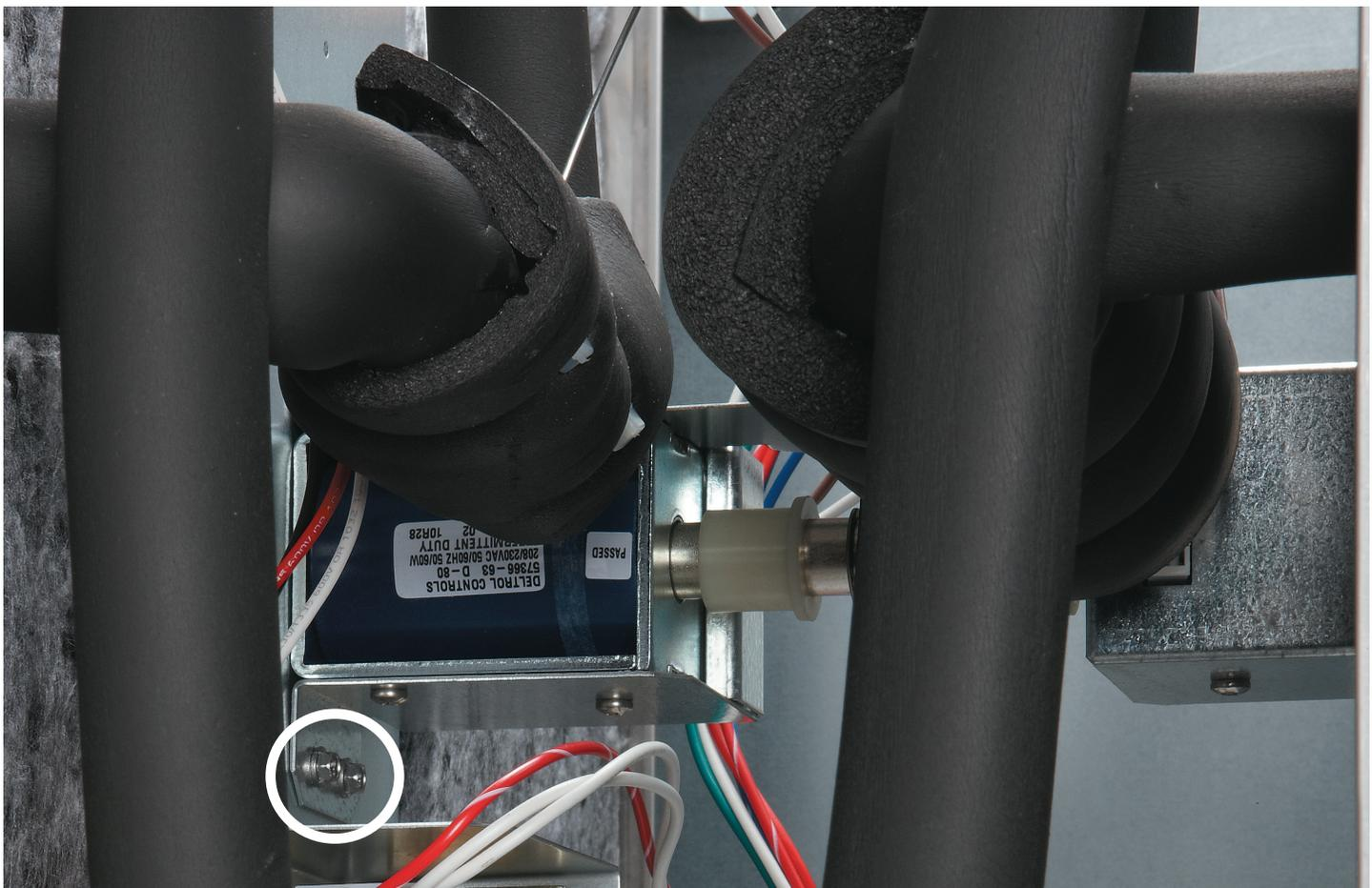
5. Remove screws holding both solenoid coils to upper bracket and remove upper bracket.
