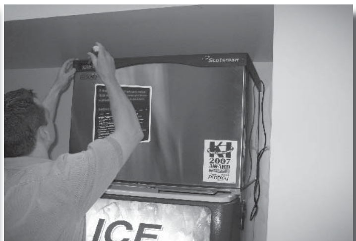
18. Re-attach front panel, discard first batch of ice.
