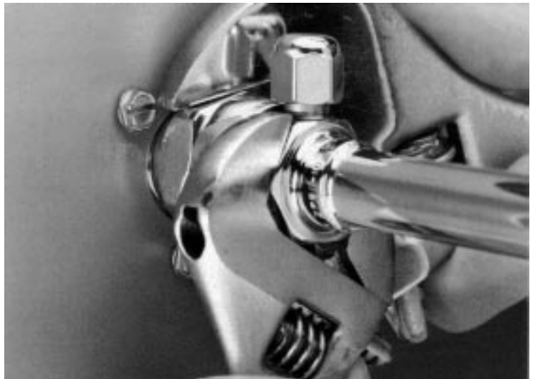
Tighten Swivel Nuts
