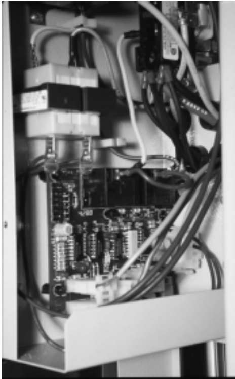
Original Control System
