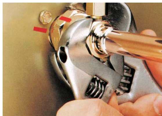
Rotate Swivel Nut 1/4 Turn More
