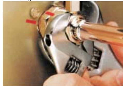
Rotate Swivel Nut 1/4 Turn More
