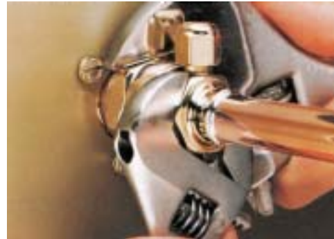
Tighten Swivel Nut
