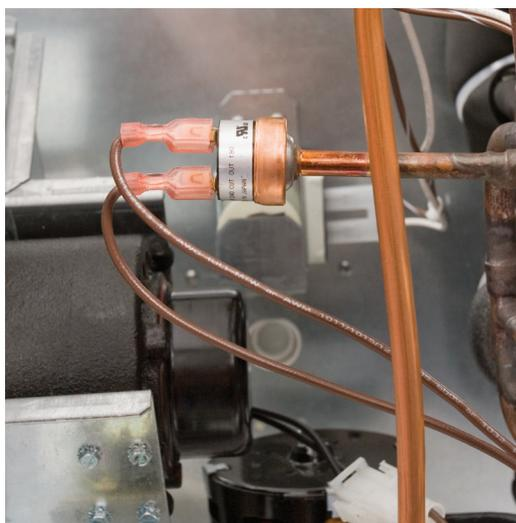
Fan Pressure Control, must CLOSE to operate fan motor.
