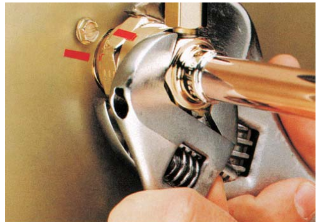
Rotate Swivel Nut ¼ Turn More
