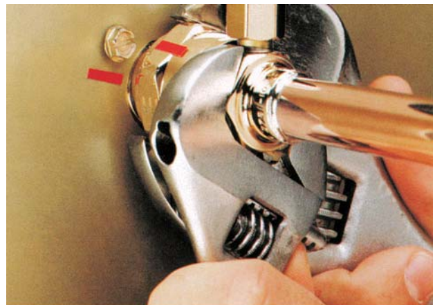
Rotate Swivel Nut ¼ Turn More
