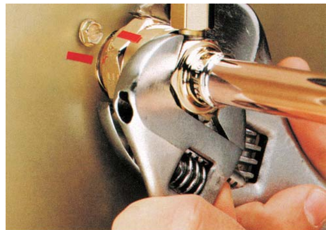
Rotate Swivel Nut ¼ Turn More
